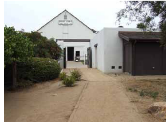
10. Sight line from garden path out (north) to Calhoun St.
