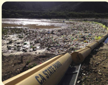
Basins capture flowing trash before it impacts the wetland and becomes marine pollutants.
